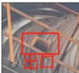
喷漆房排气筒 DA002 监测孔
