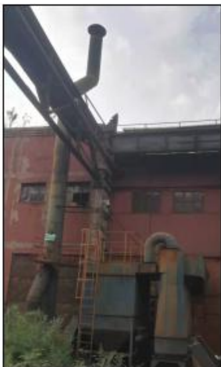
抛丸机布袋除尘器+排气筒 DA001
